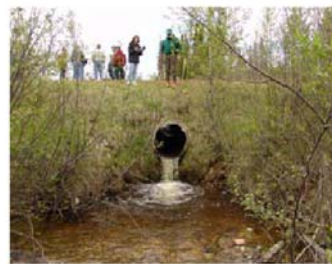
Hanging culvert on oil and gas road.
