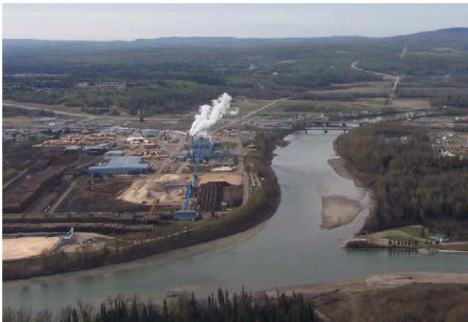
Millar Western pulp mill in the town of Whitecourt.
