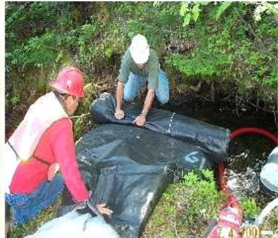
Checking for Proper Seal
