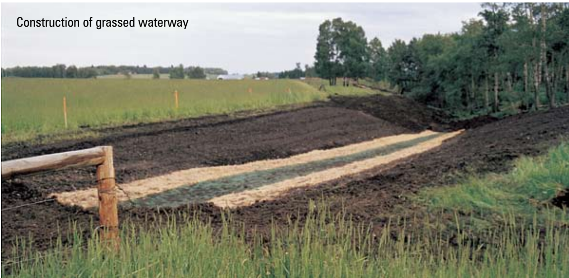
New grassed waterway
