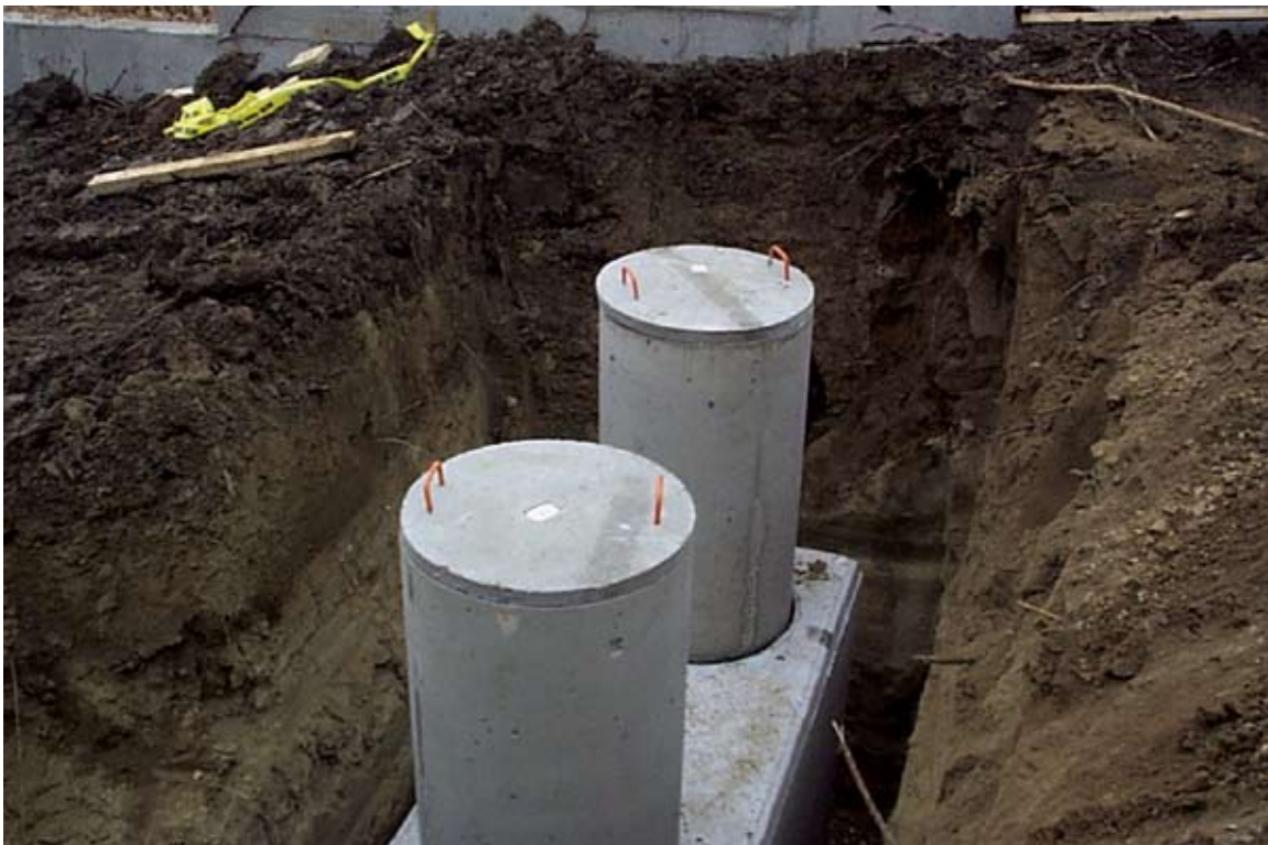
Septic tank installation — Courtesy of Safety Services, Alberta Municipal Affairs
