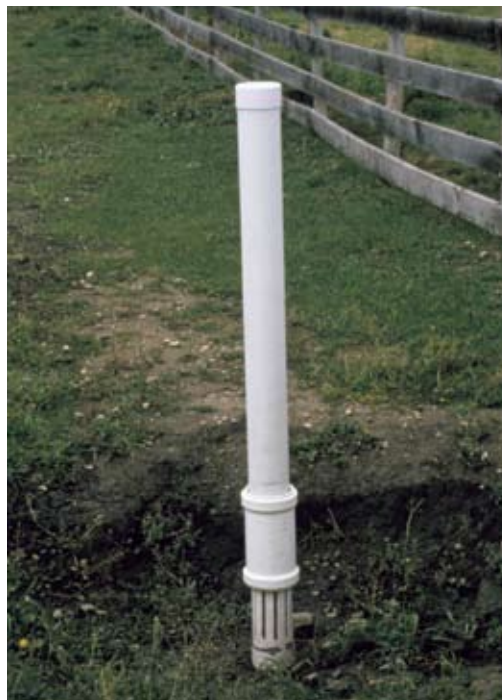
A clean water inlet pipe collects clean run-on water upslope of a livestock yard and discharges it below the yard through a drain outlet — Courtesy of AAFRD
