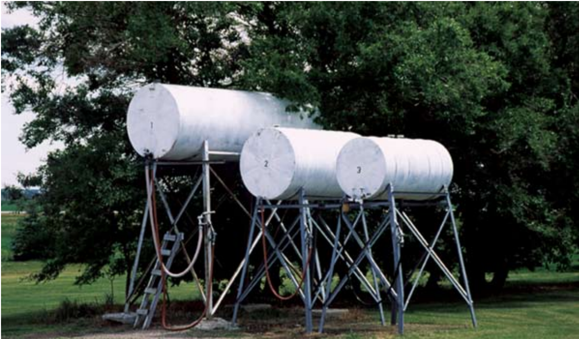
Aboveground or gravity-fed tanks located too close to trees increase fire hazards and damage from fallen trees — Courtesy of AAFRD
