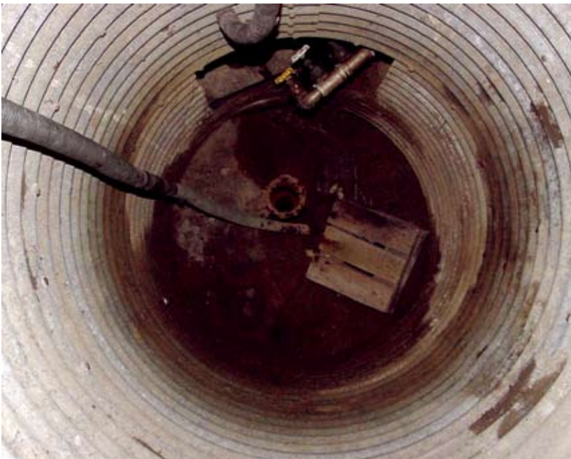
Well pits are no longer used in new well construction — Courtesy of PFRA
