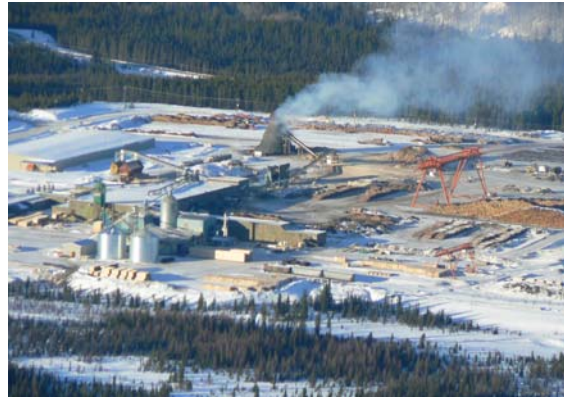
Above – Overview picture of Foothills Forest Products facility and site.
