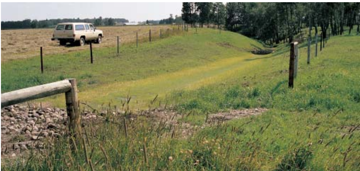
➔ Construction of a lined channel.
