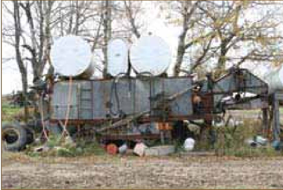
Figure 21: Example of an inadequate fuel storage system Photo courtesy of Alberta Environmental Farm Plan Company, 2006
