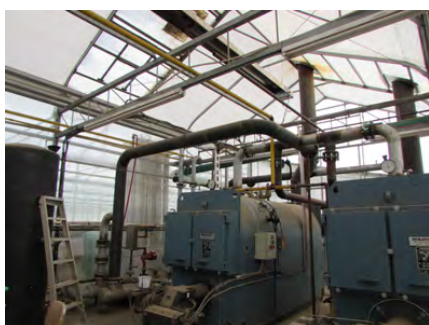
Insulate hot water pipes in areas where heat is not required, such as mechanical areas and supply/return headers within the greenhouse space.
