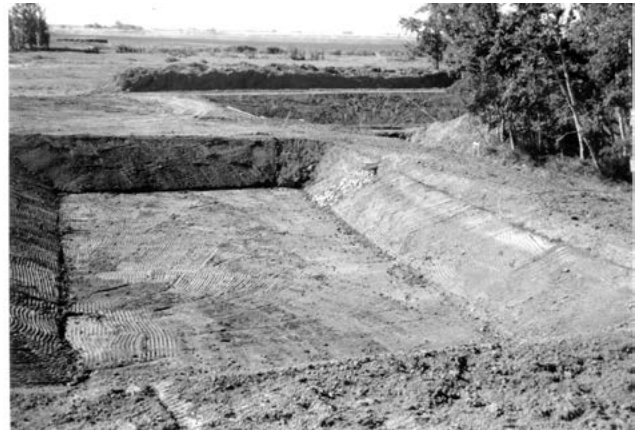
Figure 1. Typical dugout construction
