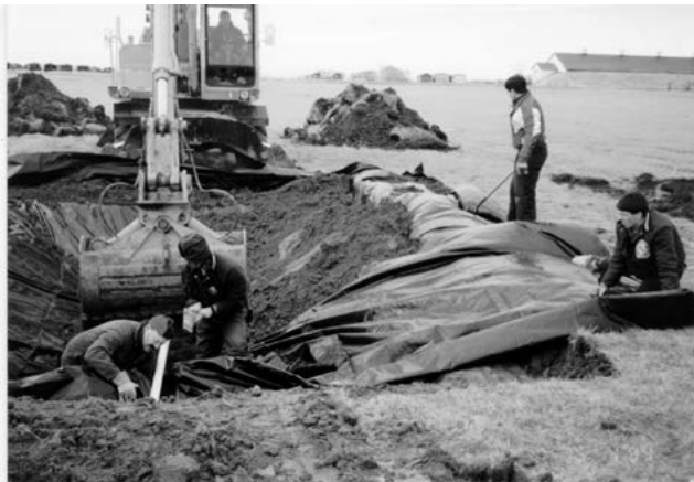
Figure 2. Installing and backfilling plastic liner
