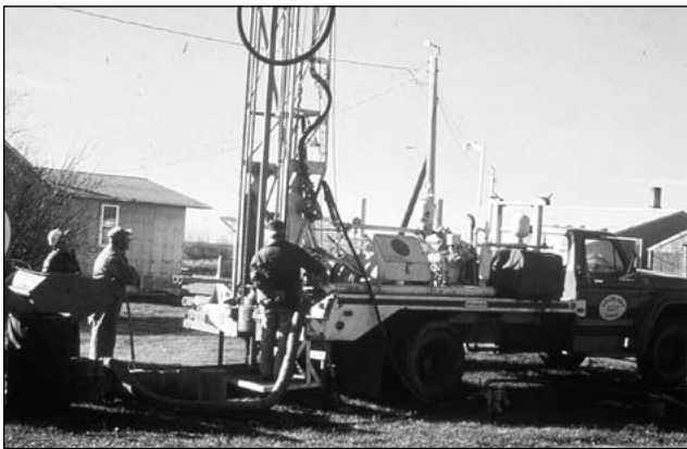
Figure 6. Test drilling to locate groundwater aquifers
