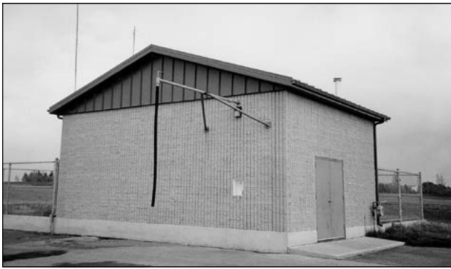
Figure 5. Tank loading facilities
