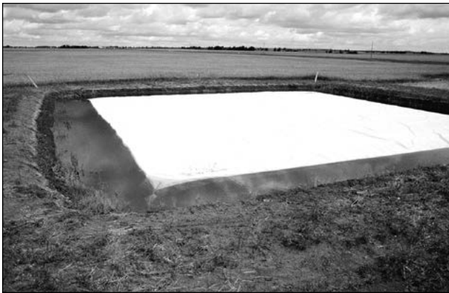
Figure 4. Plastic cover to reduce dugout evaporation losses
