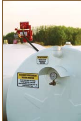
Figure 12: Double wall vacuum monitoring gauge Photo courtesy of the Alberta Environmental Farm Plan, 2006
