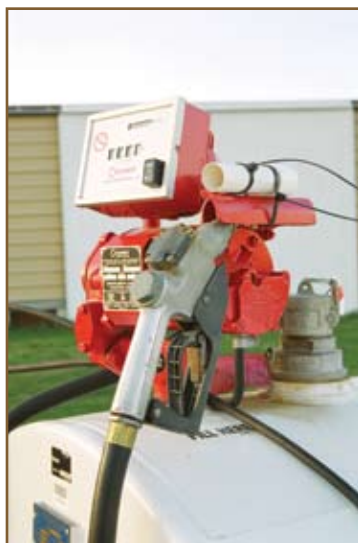
Figure 20: ULC approved pump and meter
