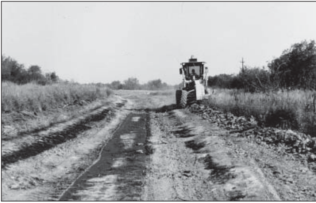
Figure 6. Road graders are useful in removing of topsoil from construction areas, repairing gullies and constructing waterways.
