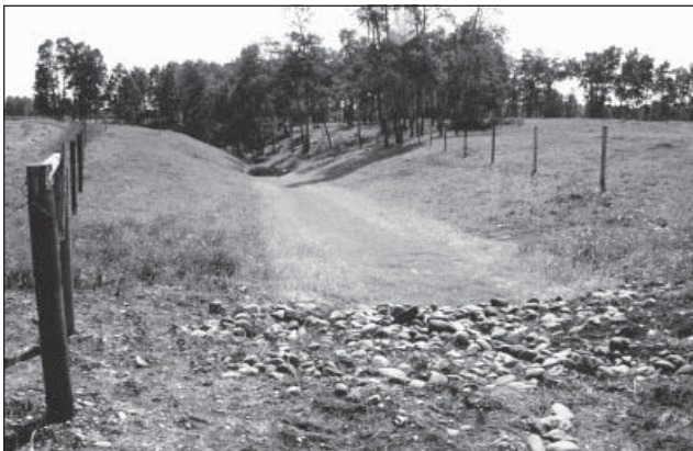
Figure 5. The North American Green P300 mat provides permanent erosion protection of steep channels carrying large amount of water.
