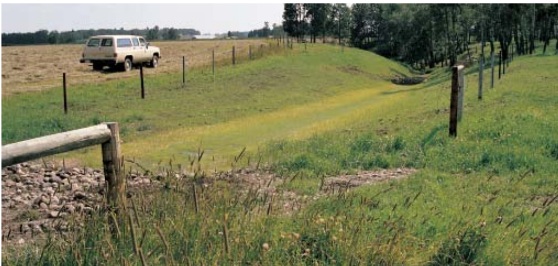
➔ Construction of a lined channel.
