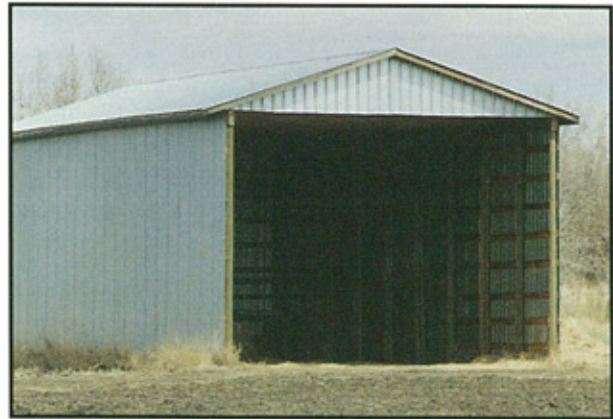
Figure 34. Pole hay shed with full walls of metal sheeting
