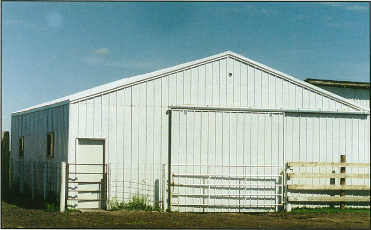
Figure 13. Straight wall metal clad stable
