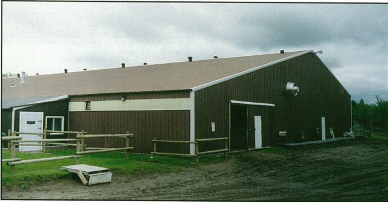
Figure 60. Metal clad arena with stalls attached to one side – note ventilation turbines and natural light strip
